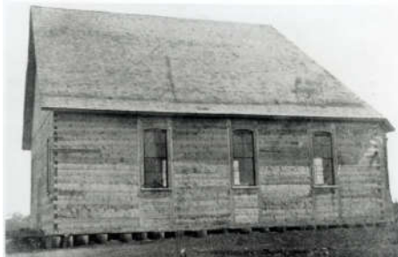
Bruderheim Church before basement addition
