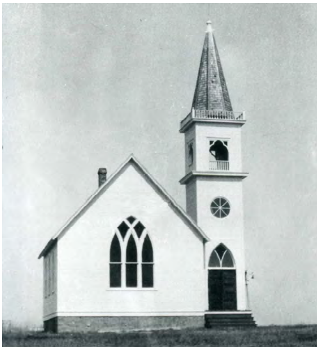
The Pleasant Point Moravian Church was built in 1910 and had a growing membership of 60 by 1918.
